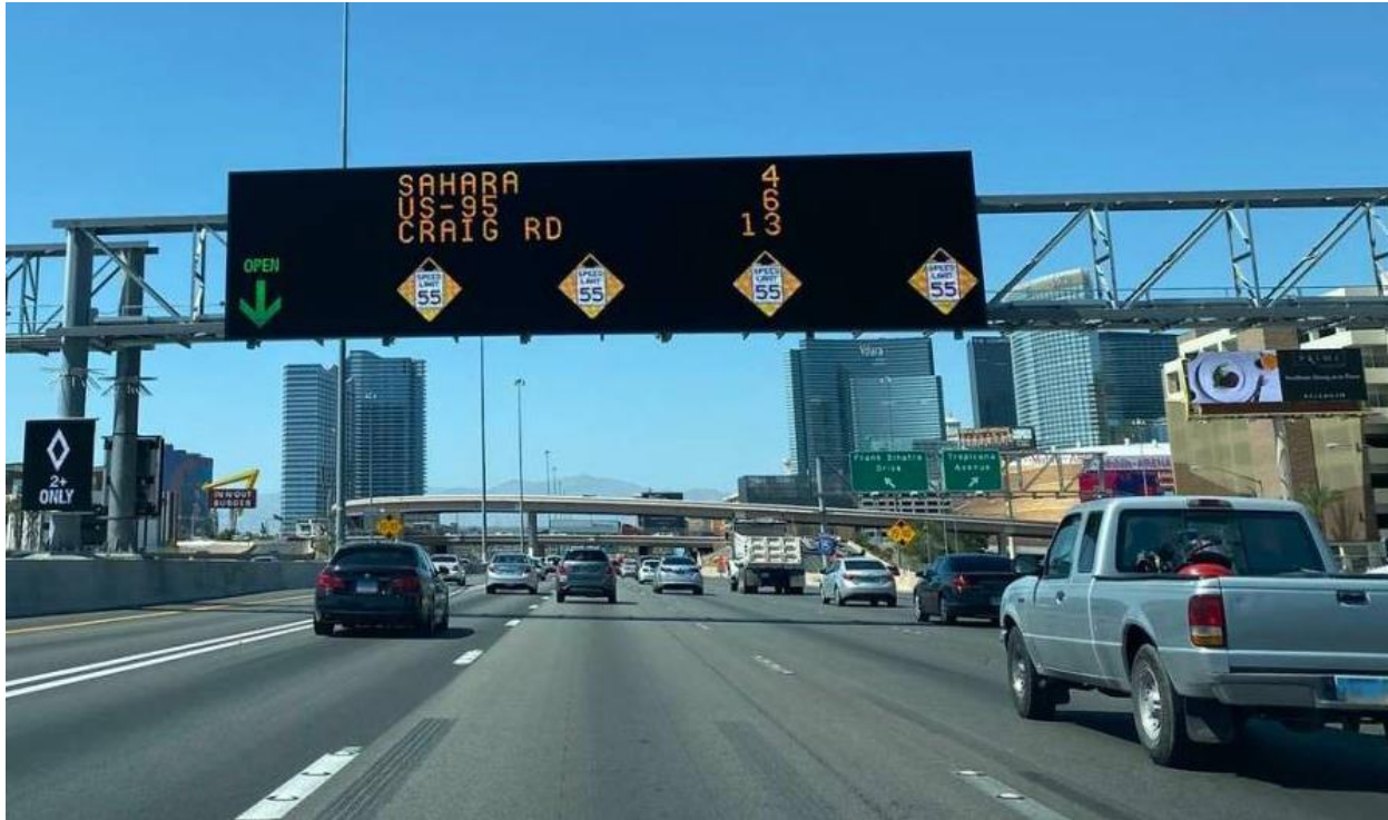
Project NEON, Nevada DOT
