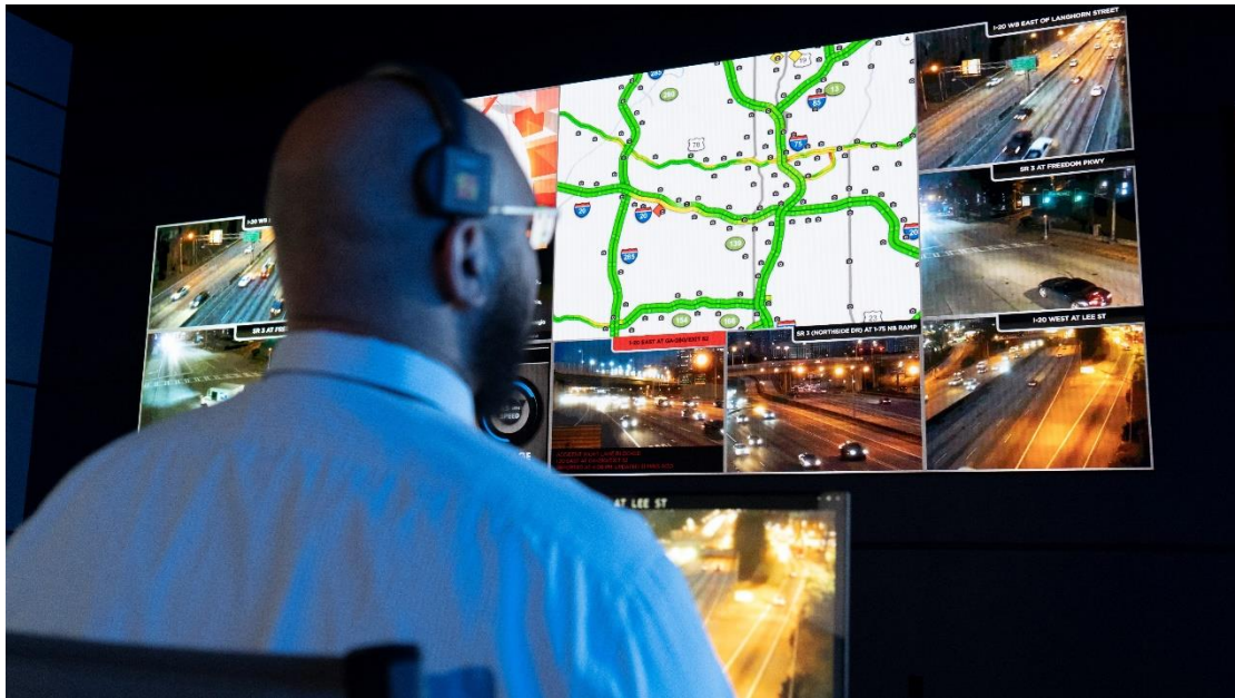
Traffic Management Center – video wall
